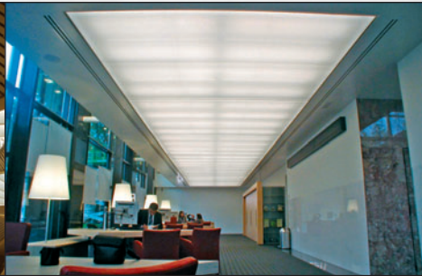
ILLUMINATED SUSPENDED CEILING
